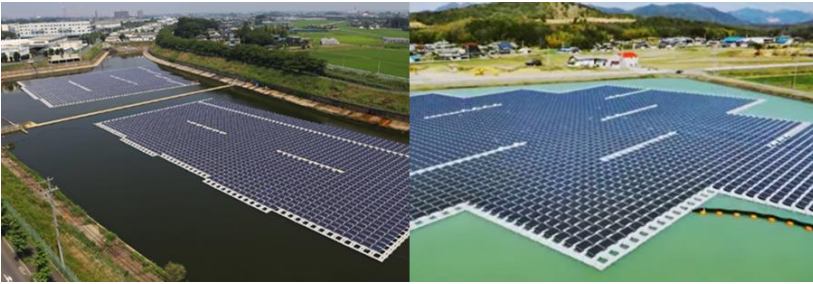
Figure 16: 1.2 MW p floating PV system at the Okegawa (left) and 1.7 MW p Hyogo (right) prefectures in Japan (NIKKEI, 2013; TECHXPLORE, 2015).
