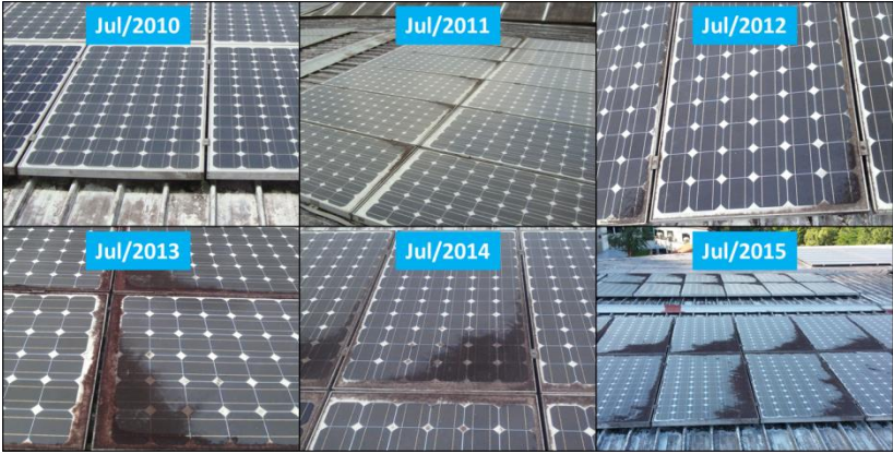
Figure 60: Progression of soiling accumulation in an unmaintained PV system due to a flat tilt angle (source: SERIS).
