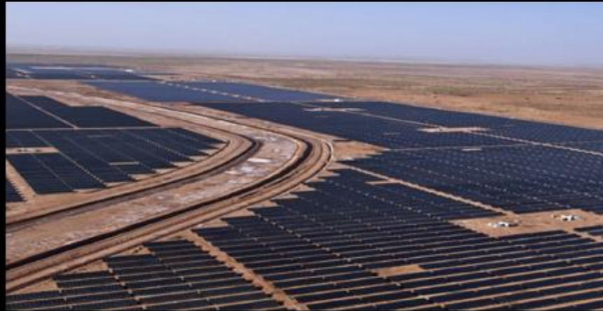
Gurjarat Solar Park Facility India (Several Locations) 857 MW (2015)
