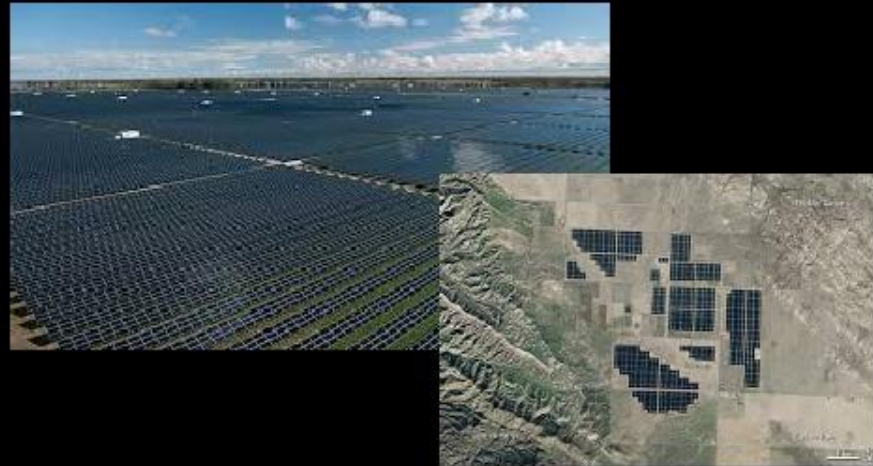
Topaz Solar Farm California, USA 550 MW (2014)
