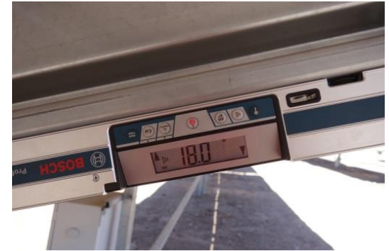
Verification of solar tracker angle
